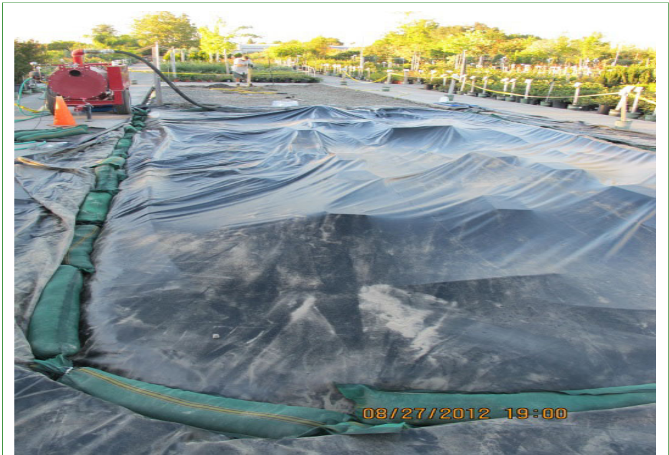
Figure 12-1-3 Tarp with Sand Snakes in Place to Secure Edges
