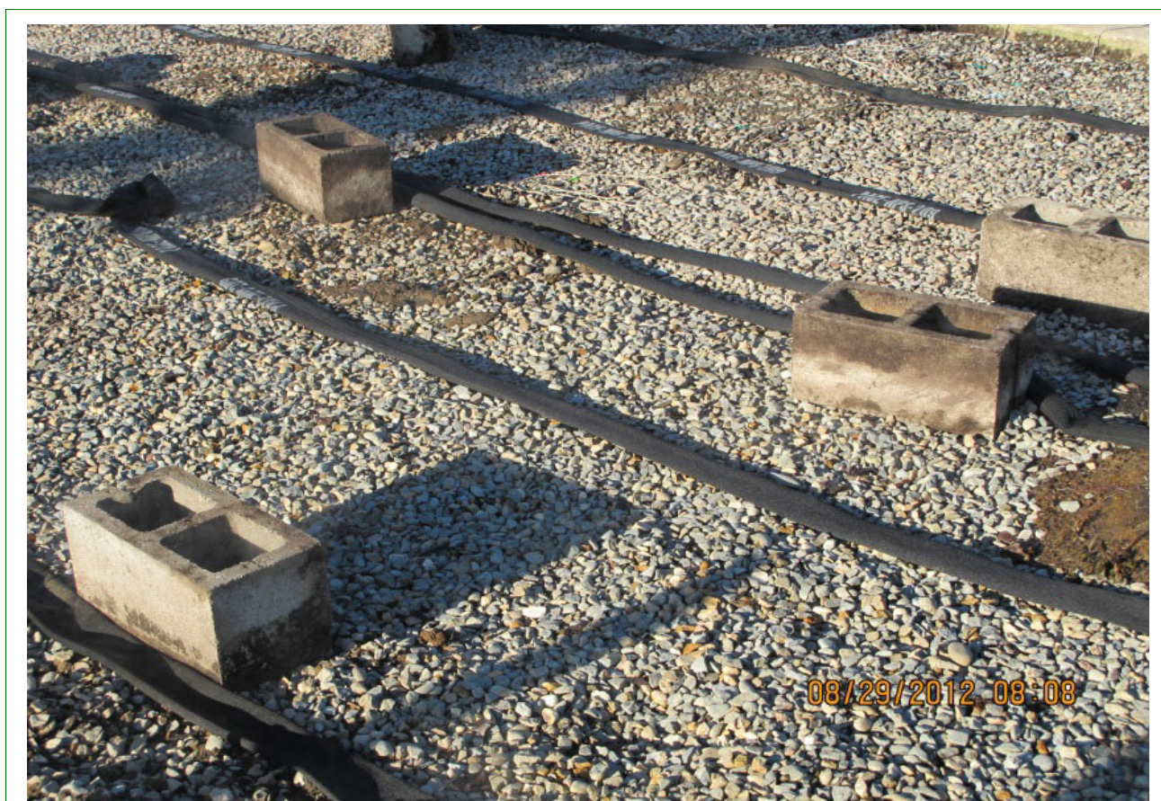
Figure 12-1-2 Concrete Blocks Used to Support Tarp from Surface to Allow Steam Distribution from Steam Sock
