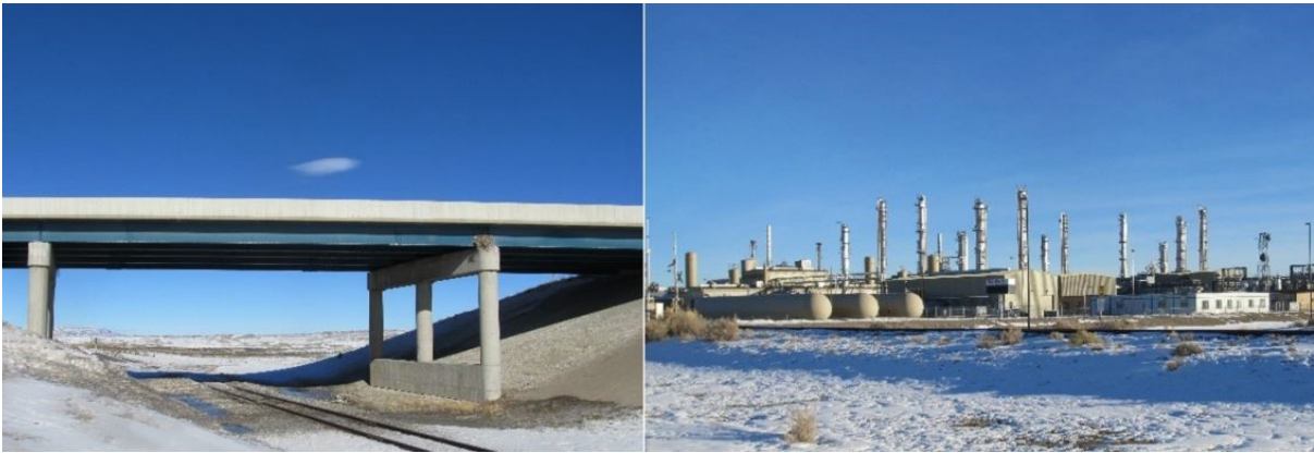
Figure 2. Ravens have been documented roosting on artificial structures, such as overpasses and heated industrial plants.
