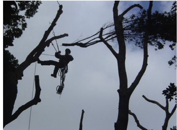
Fig. 1. A recently trimmed portion of the canopy in a Trim plot in the Canopy Trimming Experiment, Puerto Rico. Note the clean cuts made by the arborist where the branches narrow to 10 cm diameter. Photograph by A.B. Shiels.
