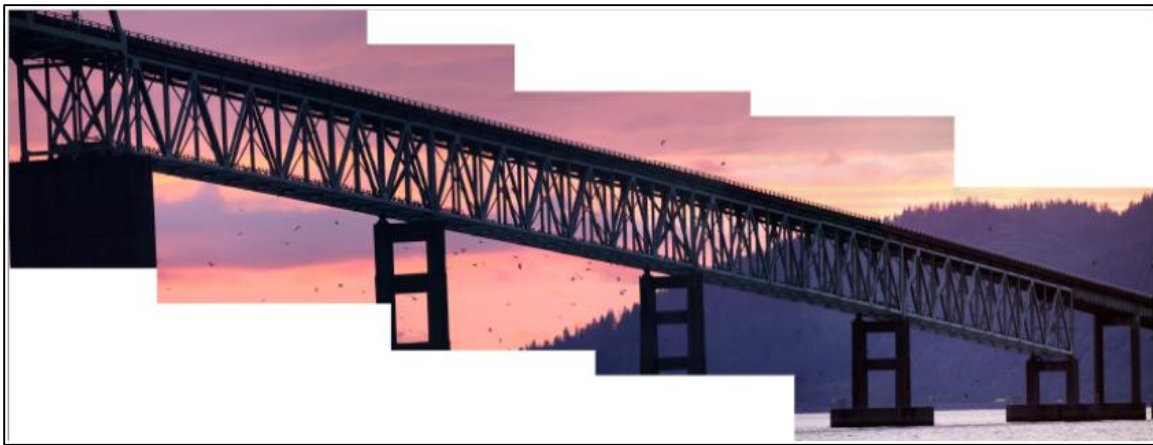
FIGURE 4-18. Steel truss section of “Bent 164” on the Astoria-Megler Bridge that is most used by DCCOs.
