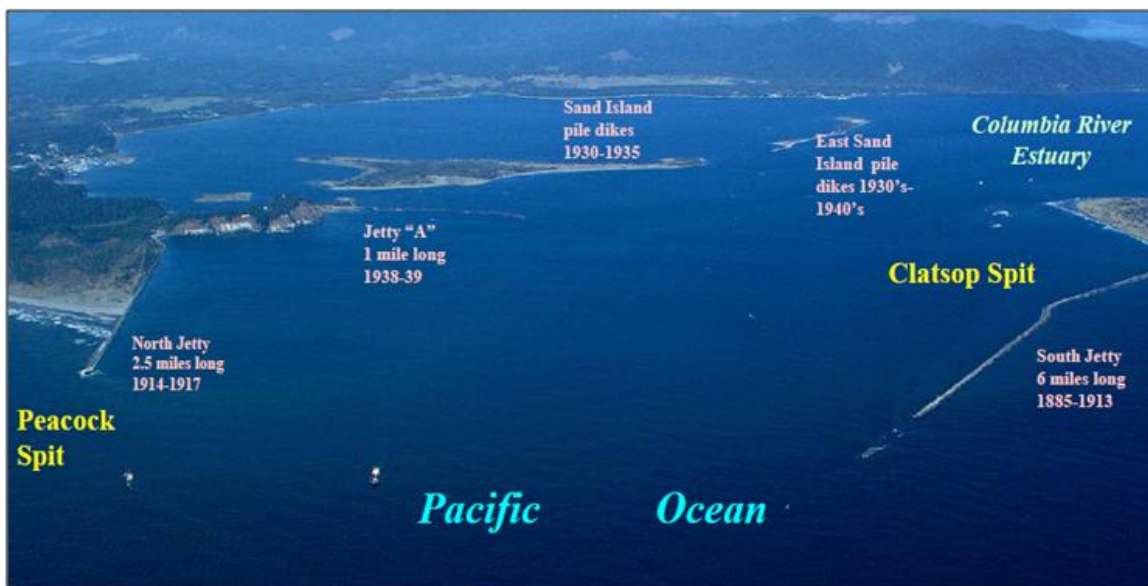
FIGURE 4-19. Mouth of the Columbia River jetty system.
