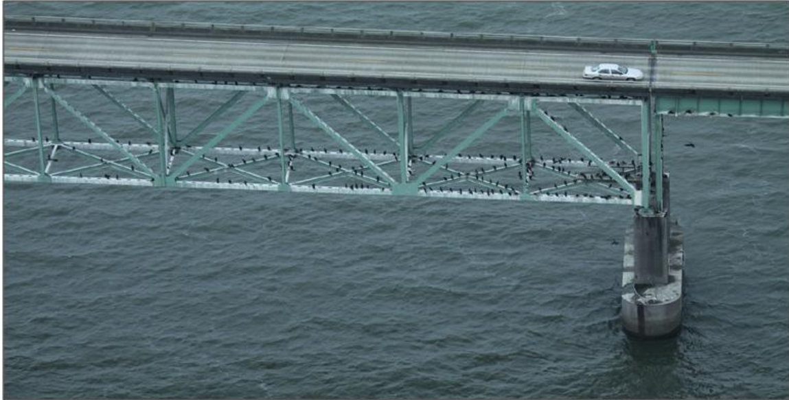
FIGURE 2-2. DCCOs using Astoria-Megler Bridge in 2012.
