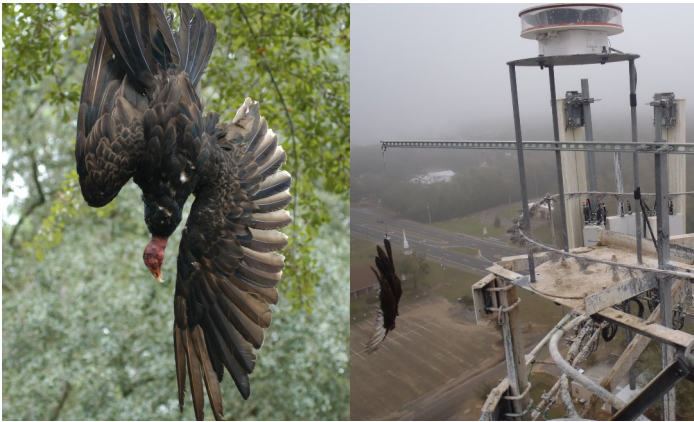
Figure 7. Installation of an effigy is effective for dispersing a vulture roost.
