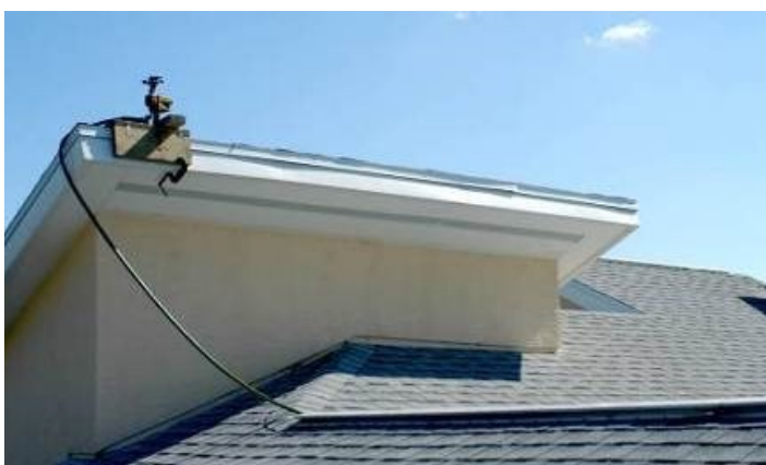
Figure 10. Motion-activated sprinklers are effective for scaring vultures from rooftops, boat docks, and other places with access to a source of pressurized water.
