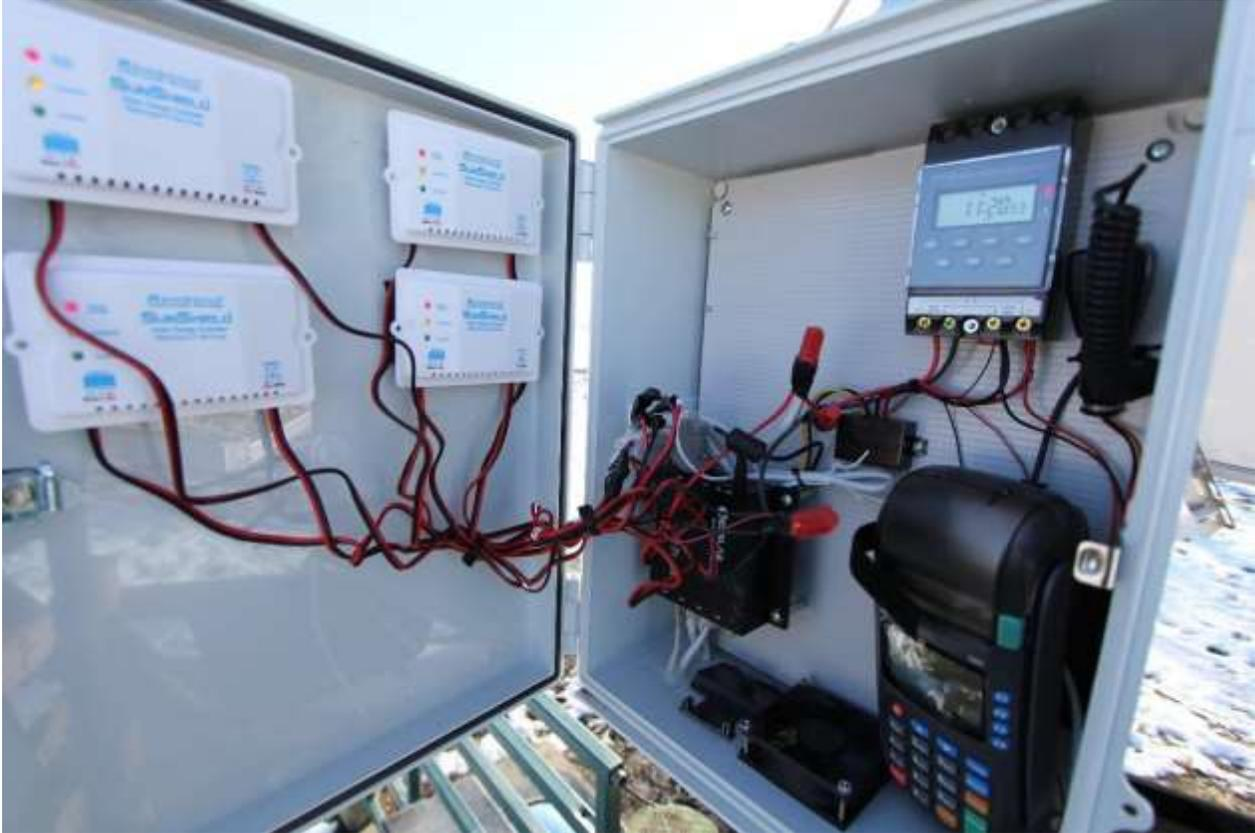
**Figure 4.** Contents of UHF RFID read point (AniMonitor, division of Hana Micron America; Milpitas, CA), which was a solar powered unit installed at the MSU Beef Cow/Calf Teaching and Research Center. Original solar charge controller was replaced with 4 solar charge controllers (Sunshield 12V 8A, Ramdsond, Detroit, MI), shown on left. Remote wireless Internet connectivity was provided by an Arymesh area network (Ayrstone Productivity, LLC, North Oaks, MN).
