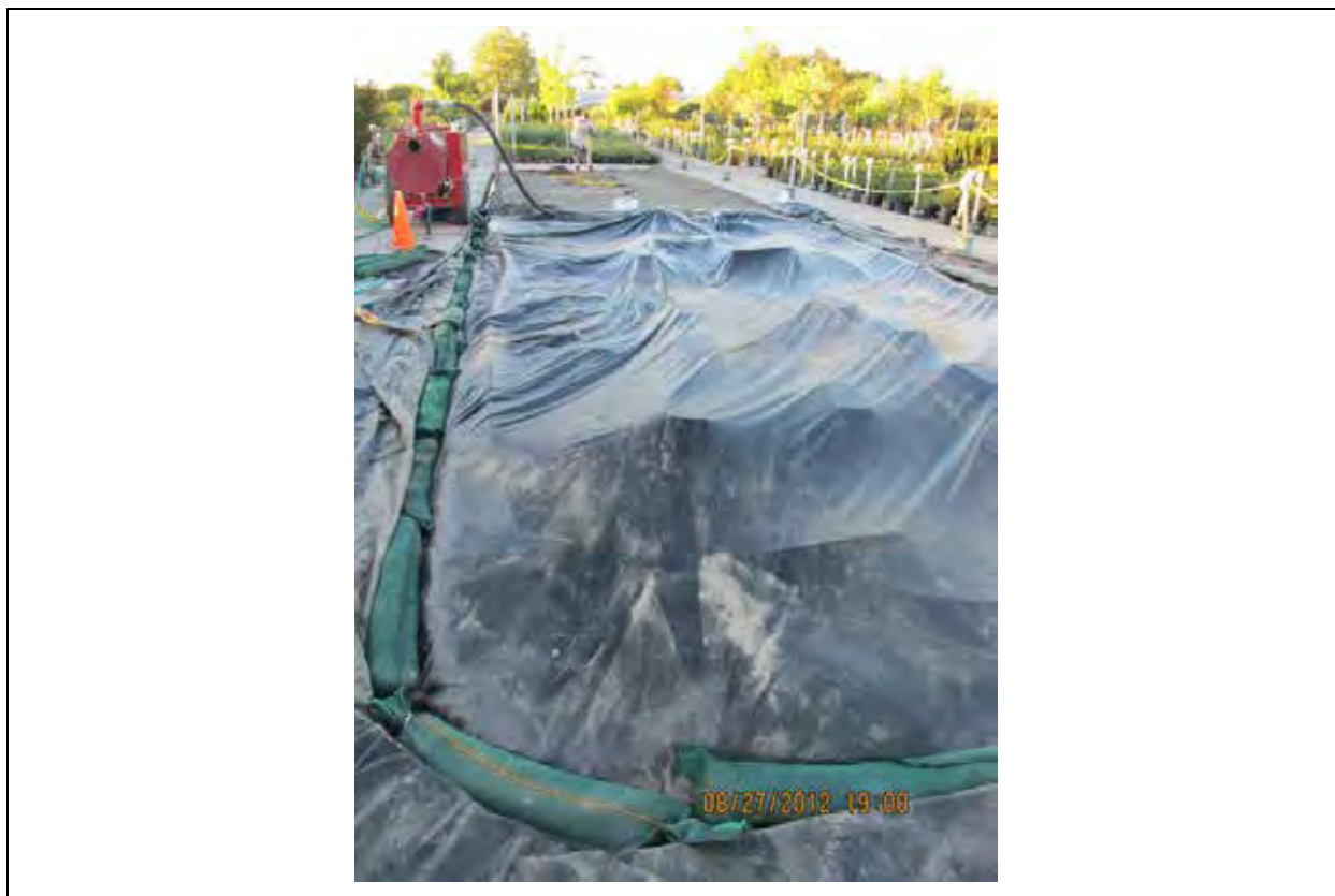
Figure 14-3 Tarp with Sand Snakes in Place to Secure Edges
