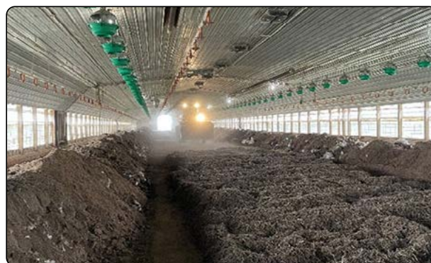
Clearing the work area
