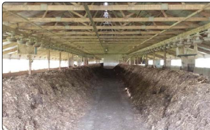
Pole house with 2 windrows (photo by Josh Payne)
