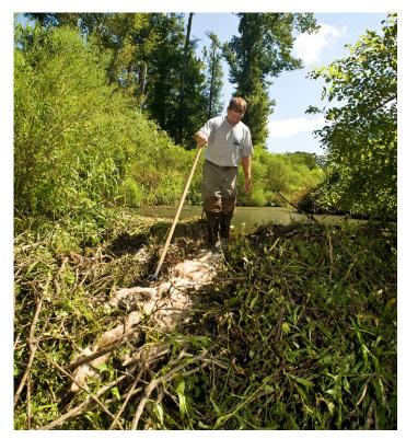
Figure 4. Damage associated with flooding by beavers generally occurs where beavers dam streams or plug culverts. Mechanical removal of dam material often is used to seek immediate results.
