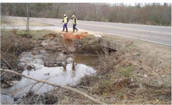
Figure 3. Beaver damage and the collapse of beaver dams can lead to structural damage of roadways and blocked culverts.
