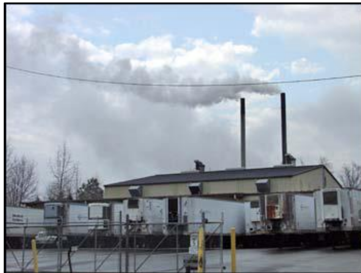
Figure 1. Off-site Incineration Facility
