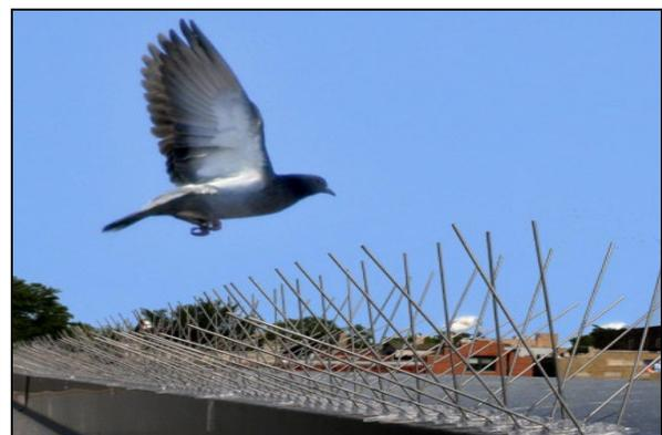
Figure 2. Example of an anti-perching device (e.g., Nixilite<sup>®</sup>) installed on a ledge to keep pigeons from landing.
