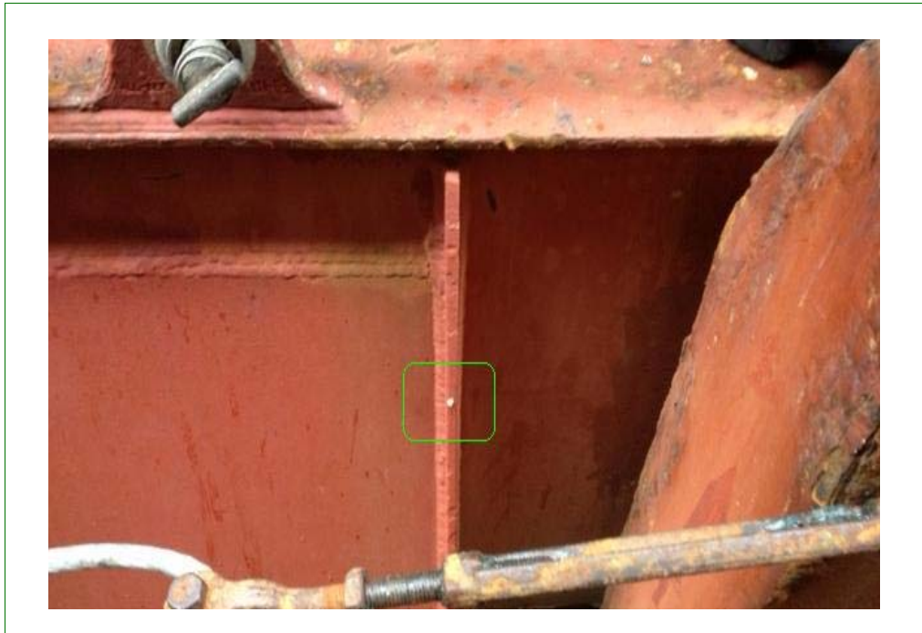
Figure 2 AGM Eggs Found Between Two Bays on a Support Beam Near a Cargo Hold Opening
