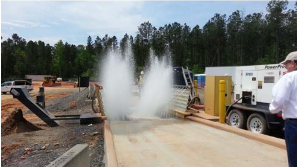
Figure 1. Water jets at Earnhardt Grading Undercarriage and Wheel Wash in Ft. Mill, SC.
