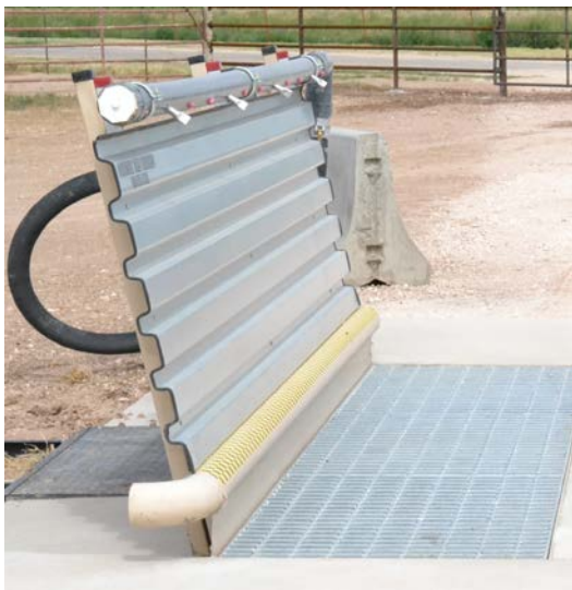
Figure 5. Left: To provide more water from beneath the vehicles, nozzles on the side wash were removed and replaced with plugs. Right: The installation in South Carolina with all side nozzles operational. To add the central channel required either adding another pump and changing the electrical requirement or diverting water from the side wash to the bottom. The feedyard manager preferred the latter.
