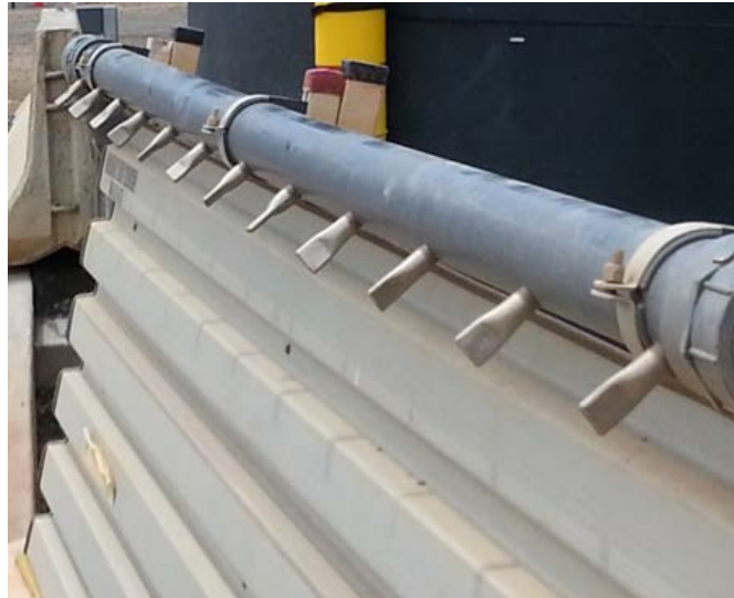
Figure 5. Left: To provide more water from beneath the vehicles, nozzles on the side wash were removed and replaced with plugs. Right: The installation in South Carolina with all side nozzles operational. To add the central channel required either adding another pump and changing the electrical requirement or diverting water from the side wash to the bottom. The feedyard manager preferred the latter.
