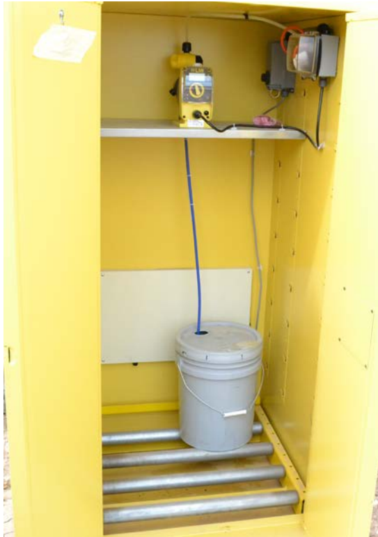
Figure 7. Waste discharge point. Material is discharged with 2% to 3% moisture content.
