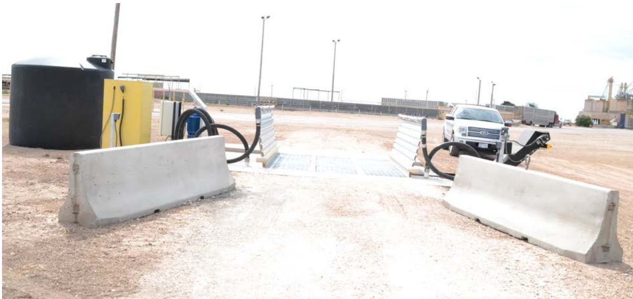
Figure 5. Left: To provide more water from beneath the vehicles, nozzles on the side wash were removed and replaced with plugs. Right: The installation in South Carolina with all side nozzles operational. To add the central channel required either adding another pump and changing the electrical requirement or diverting water from the side wash to the bottom. The feedyard manager preferred the latter.
