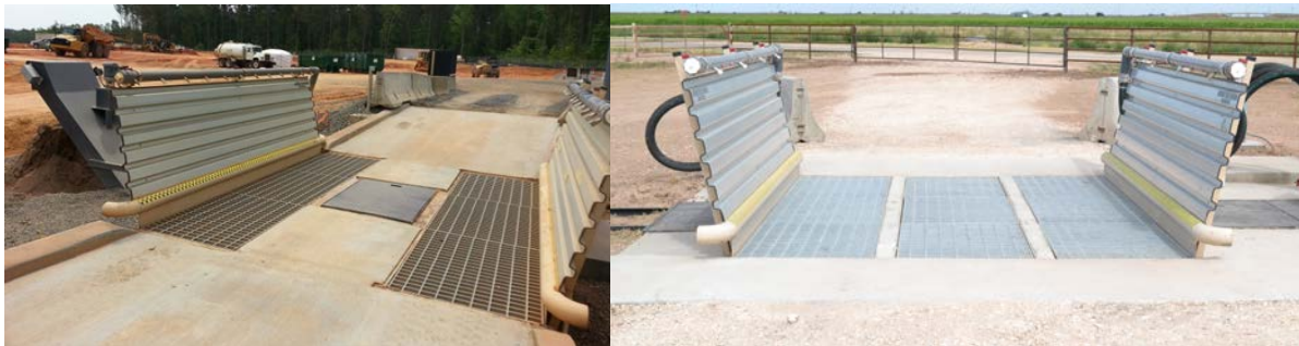
Figure 2. Left: STB 30 in FT. Mill, SC. Notice there is no central channel. Right: Unit install in Texas with central channel. The central channel was requested by the feed yard manager.
