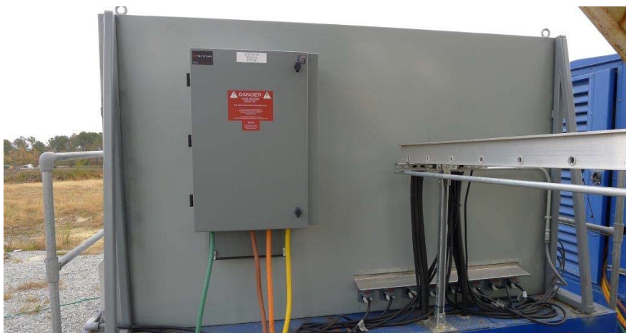
Figure 13. Generator Docking Station
