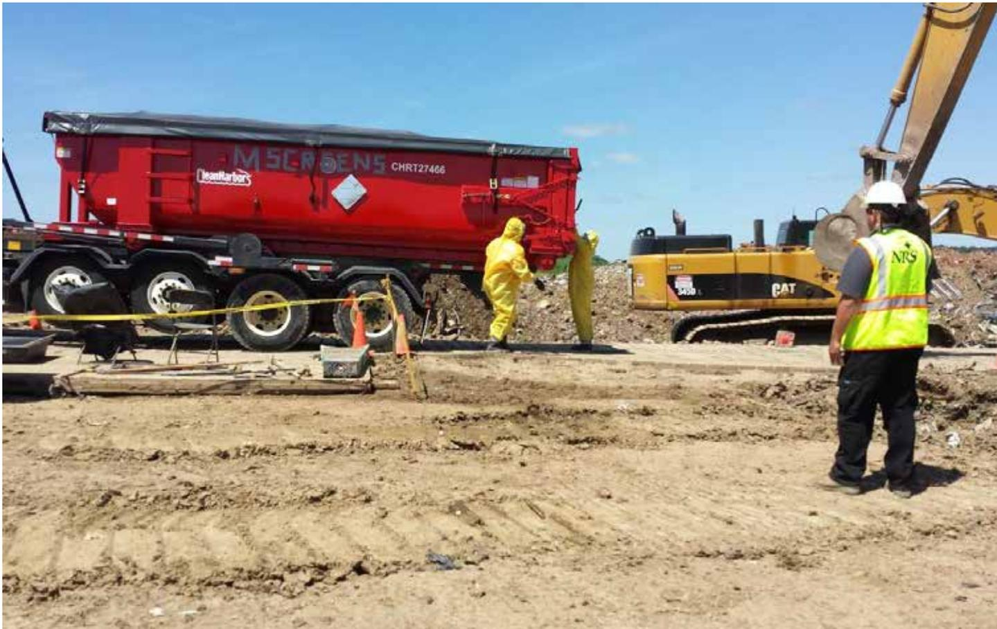
Preparing to dispose of load. Excavator and delivery truck personnel communicate using a series of honks.
