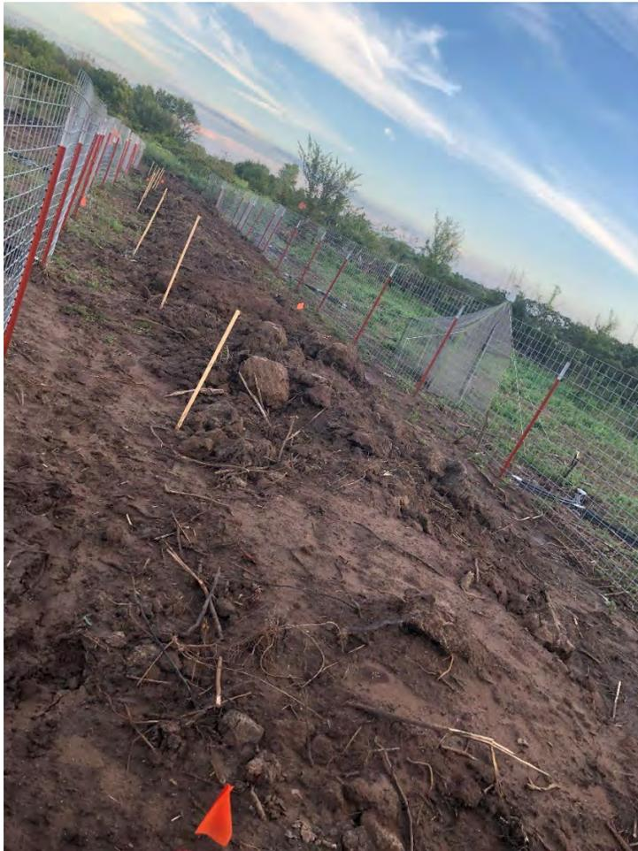
Figure 411. Animal mortality trench after animal and trap placement
