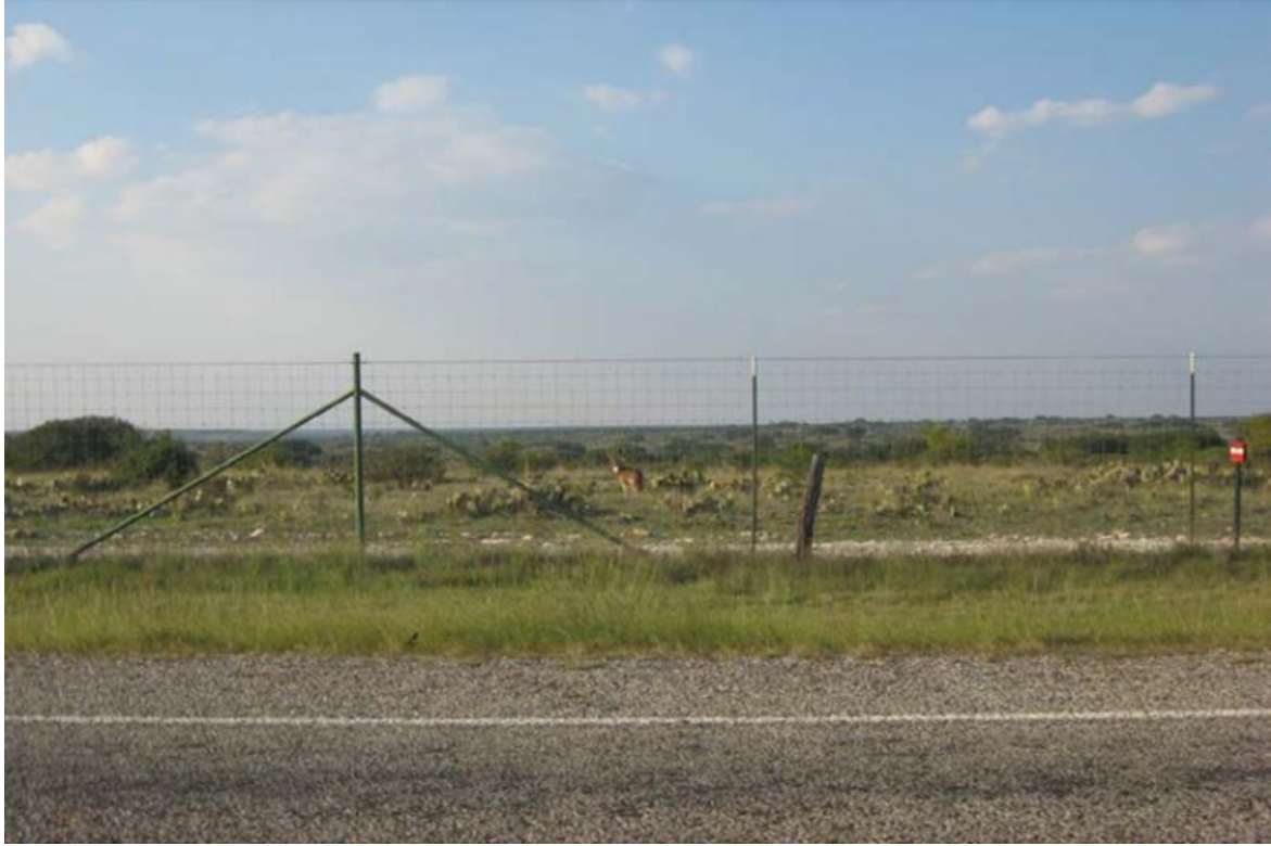
Figure 5. Example of wire-knot game fencing
