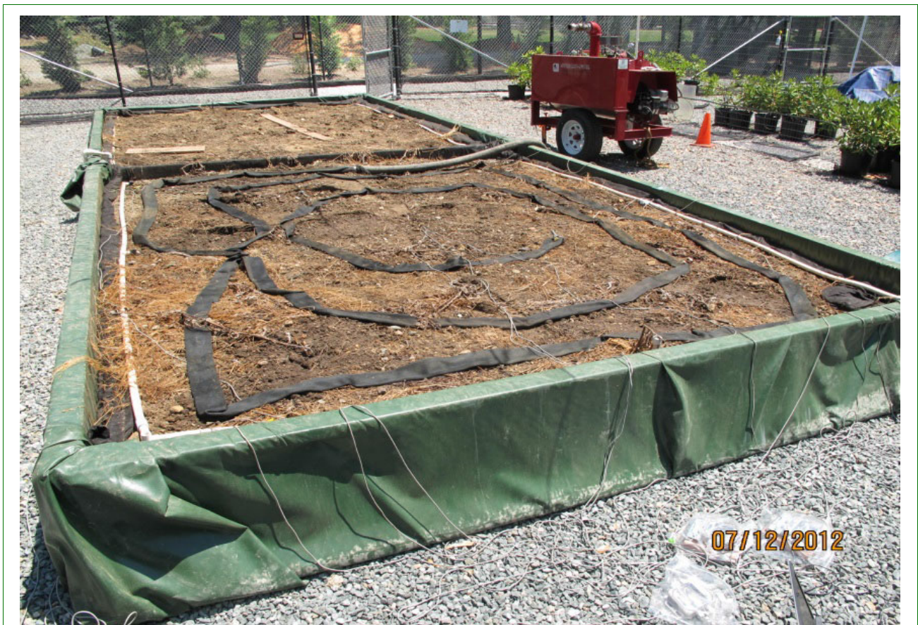
Figure 12-1-1 Steam Sock in Place on Soil Surface
