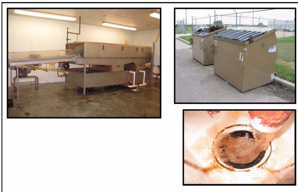
PHOTO 22: Haringen ERF: Tower Tray Wash and Waste Disposal
