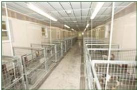
This indoor facility has sealed concrete floors and the walls are an easily cleanable surface. The ceilings have replaceable tiles.
